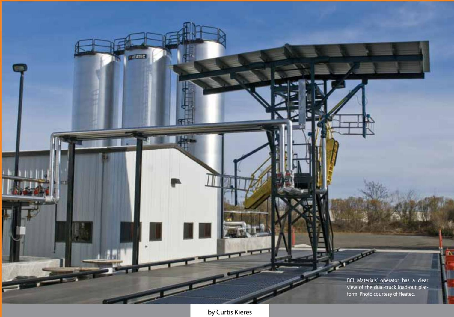
BCI Materials' operator has a clear view of the dual-truck load-out platform. Photo courtesy of Heatec.
